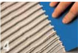
Start by making ribs in the glue with a notched spatula (6 mm for Interfix, 8 mm for Granulit and 10 mm for Murok).
