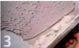
Apply the adhesive in sections of ½ m² so it doesn't dry before you fix the brick strips. Stains from spotting and spilling can then still be easily removed.
