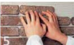
Then apply the strip in a sliding motion. Always start with the corners and mix strips from different boxes.
