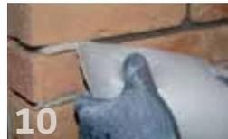
Cladding with joints: Filling joints is done with Cemix Unijoint which is mixed with water. Fill the joints using a mortar plastic bag. Keep using the same proportion of water to avoid colour variations.
