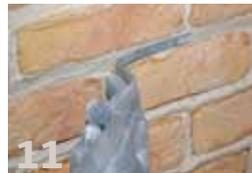
When the joint begin to harden, tighten it with a narrow trowel or simply with the wooden handle of a brush. Do not touch the joints as they are fresh and they have not sufficiently cured. If the cladding is stained by the mortar, wipe gently with a sponge soaked in water.
