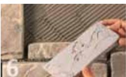
For the heavier stone products of the Murok range the installation with the back-butter technique is required. This means that the glue must be applied as well on the back of the slips as on the wall-surface.
