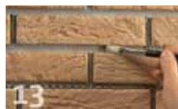
Interfix: the joints can be filled in the traditional manner. Or the Interfix glue can be stroked smooth in the joint. Do this with a damp finishing brush, such that the glue seals with the edge of the strip.
